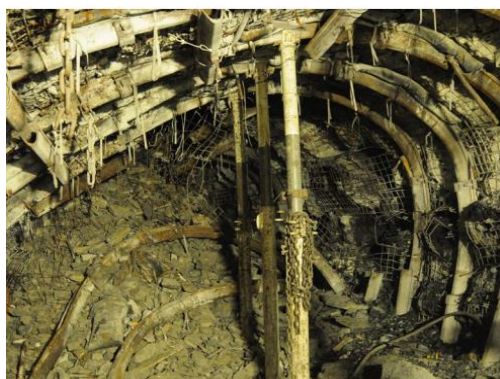
Figure 1. Recovery of iron supports along the 5-level +290 seam at Ke Chuoi Coal Mine
