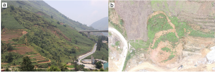
Fig. 6.2 Photo of the Mong Sen landslide (a) and the landslide site (b) in Trung Chai area
