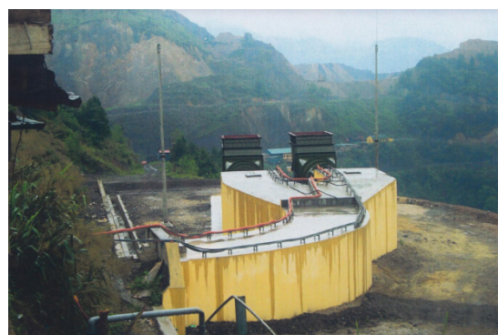
b) Trạm quạt FBCDZ-10-No3.5
