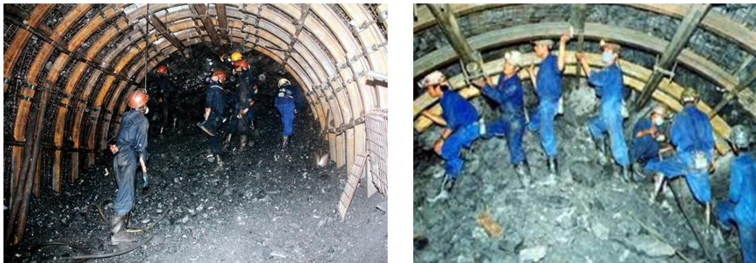
Fig. 3. Steel arch support systems in the mine tunnels
