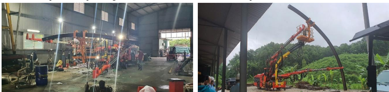
Fig. 13. Experimentally fabricated steel arch support lifting mechanism and evaluated for real performance
