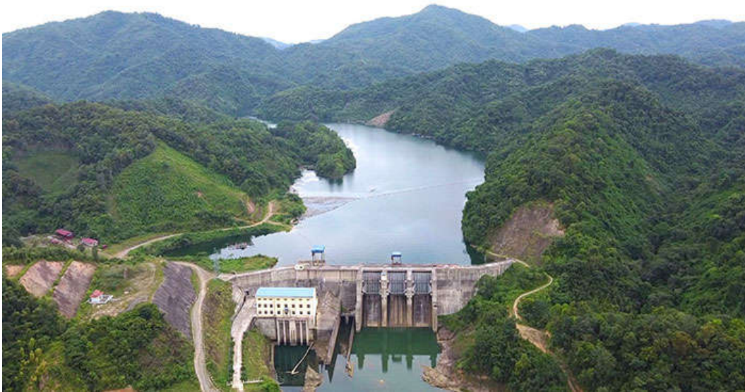
Figure 3. Thac Xang Hydroelectric Power Plant
