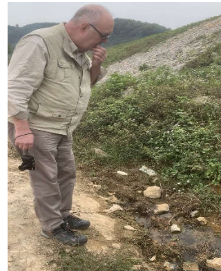
Figure 5. Field survey at a seepage point located 15 m upstream of leakage point at the downstream toe of Dap Troi Dam (18/01/2023), when the reservoir water level was low
