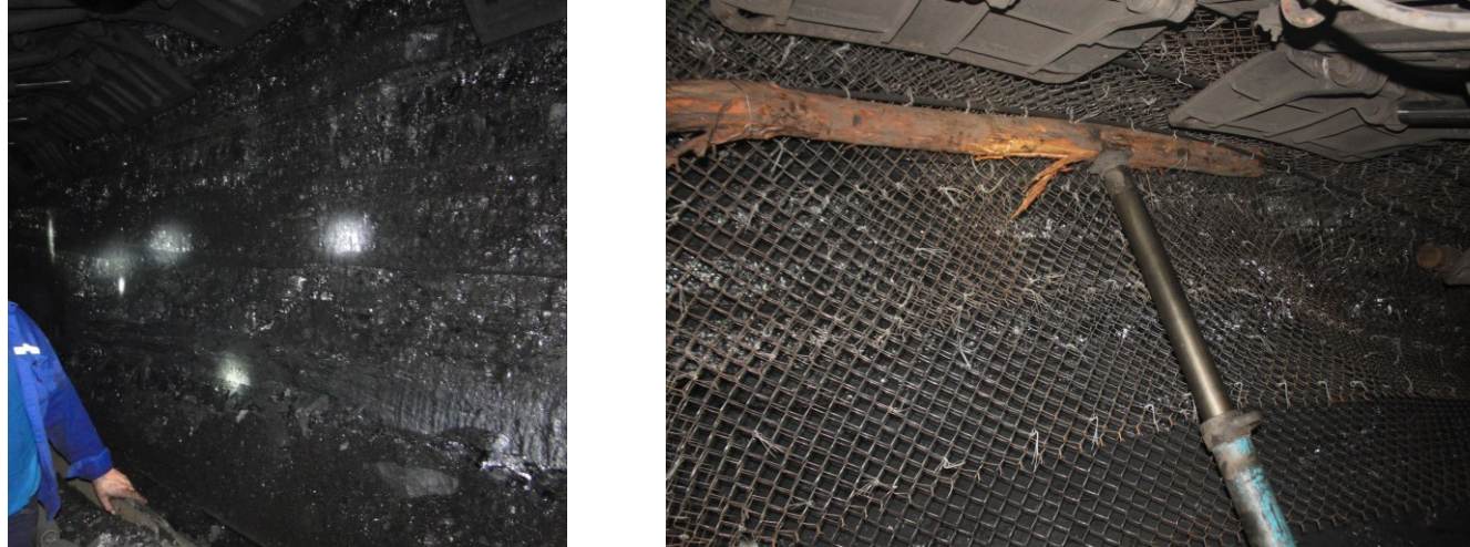
Fig. 1 Longwall face in Vang Danh coal mine, Vietnam: stability (left, no mesh) and instability (right, with mesh)
