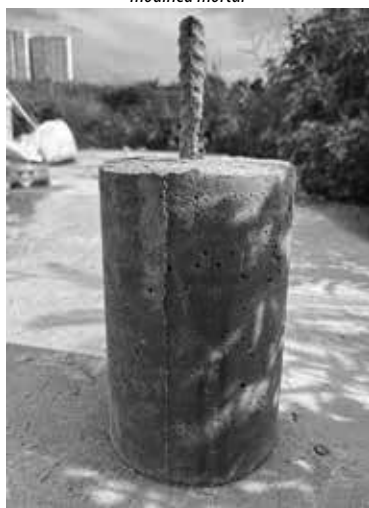
d) High-strength mortar-coated concrete sample after the corrosion test in a corrosive environment
