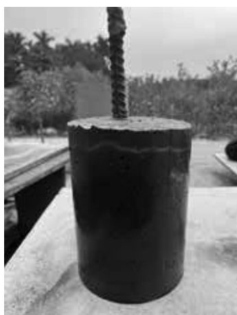
b) Sample of concrete coated with high-strength modified mortar
