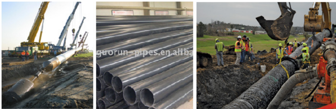
Figure 6: The pullback operation and types of pipe(s) (Source: internet)
