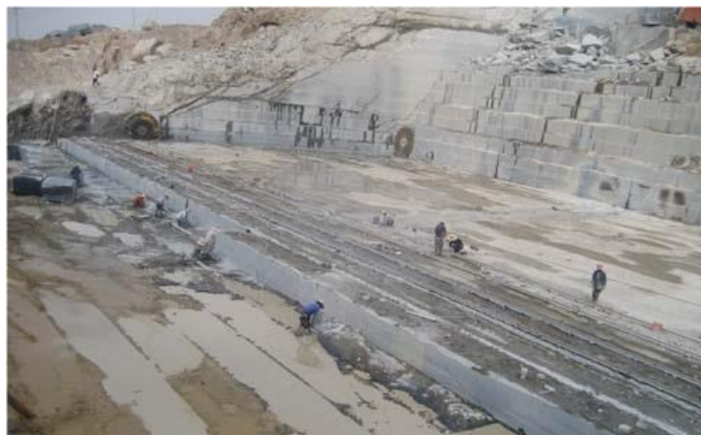
Fig. 5. Combined technology among disc sawing, diamond wire sawing and wedge is operated in a dimension stone quarry
