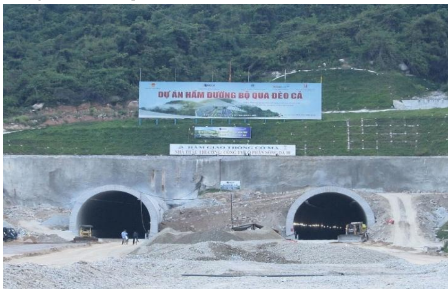
Fig. 2. Deo Ca traffic tunnel
