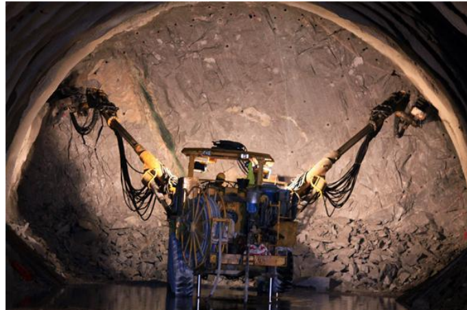
Figure 2. Deo Ca tunnel.
