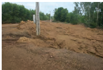
Fig 12: Tra Son Hamlet, solid waste spills over into residential areas, encroaches on roads, and affects high - voltage power lines.
