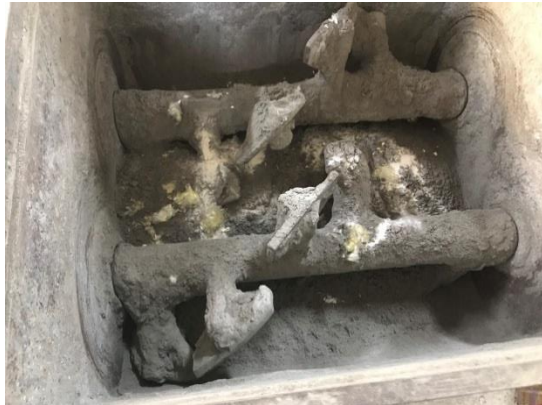
a) Preparation of concrete mixer
