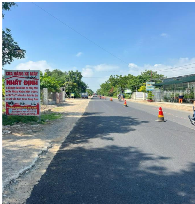
3 days after Microsurfacing
