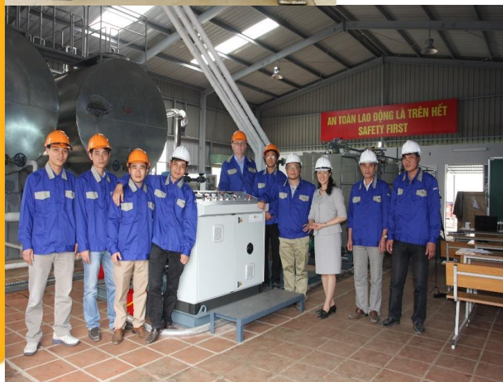
Production Line (Emulbitume- from France)- Capacity 15 t/hr.
